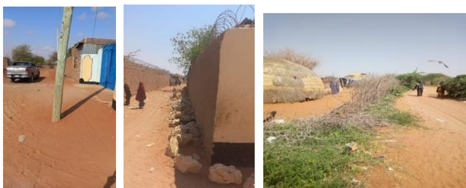
Figure 2-12: power pole, hedge and masonry wall encroachment in Godade location
