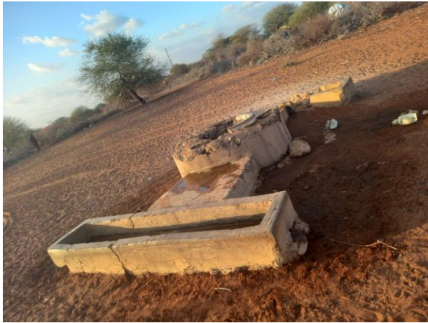
Plate 4-9: One of the community shallow well in Lambib with animal watering trough
