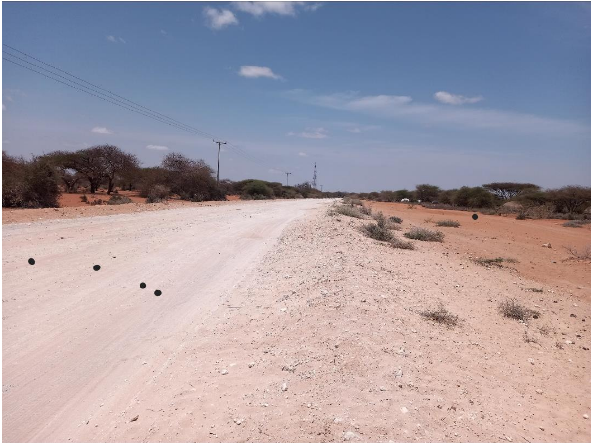
Kumbi Water Pipeline – Free from Encroachment or any community establishments
