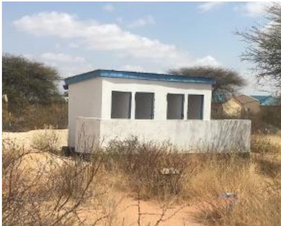
Figure 2-11: Existing Toilets at Furaha Mixed Secondary School
