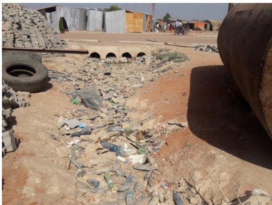
Photo Plate 1-4: Drainage channels within Wajir CBD choked with debris and solid wastes
