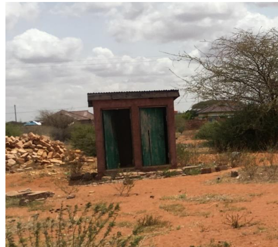
Figure 2-14: Toilet at Wagberi Mixed Secondary School
