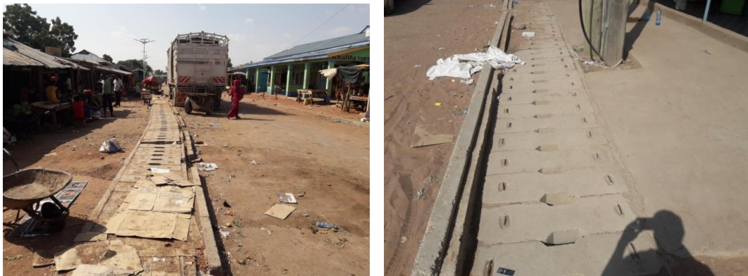
Photo Plate 1-5: closed / covered drainage channels within Wajir grocery market, these channels are encroached
