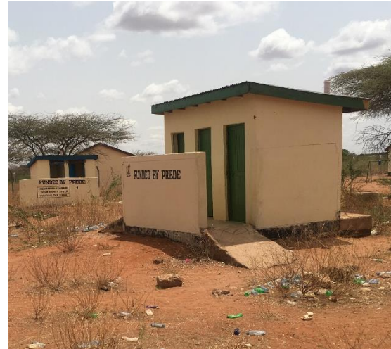
Figure 2-8: Existing Toilets in Jogbaru Primary School
