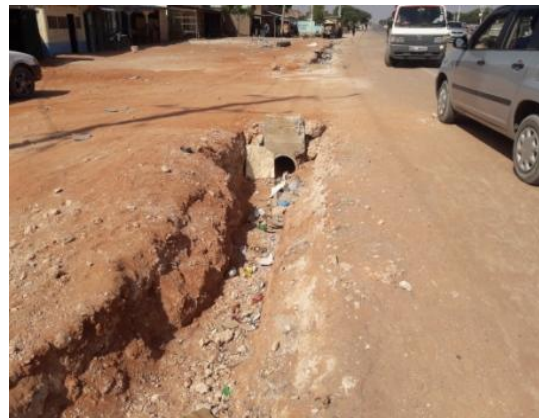
Photo Plate 1-3: Unlined Drainage channels along Wajir – Moyale Road
