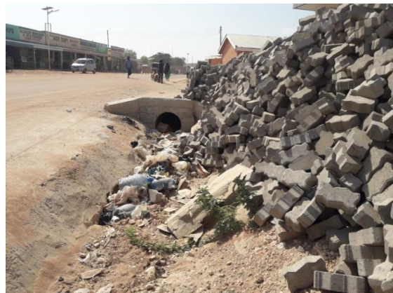
Photo Plate 1-4: Drainage channels within Wajir CBD choked with debris and solid wastes
