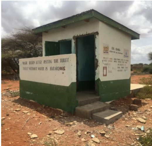
Figure 2-7: Existing Toilet with attached Septic Tank in Rahma Primary School
