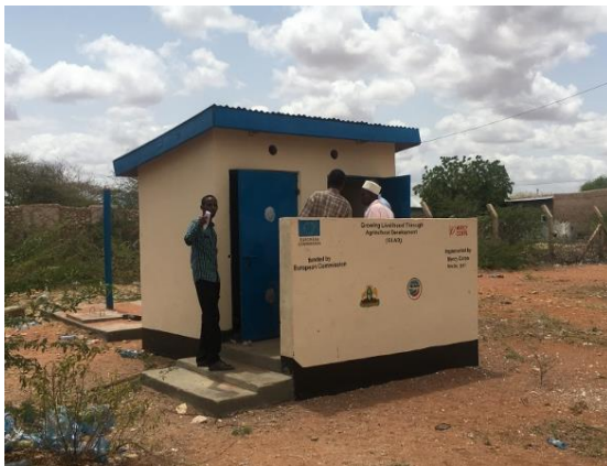
Figure 2-9: Existing Toilet with attached Septic Tank in Hothan Primary School
