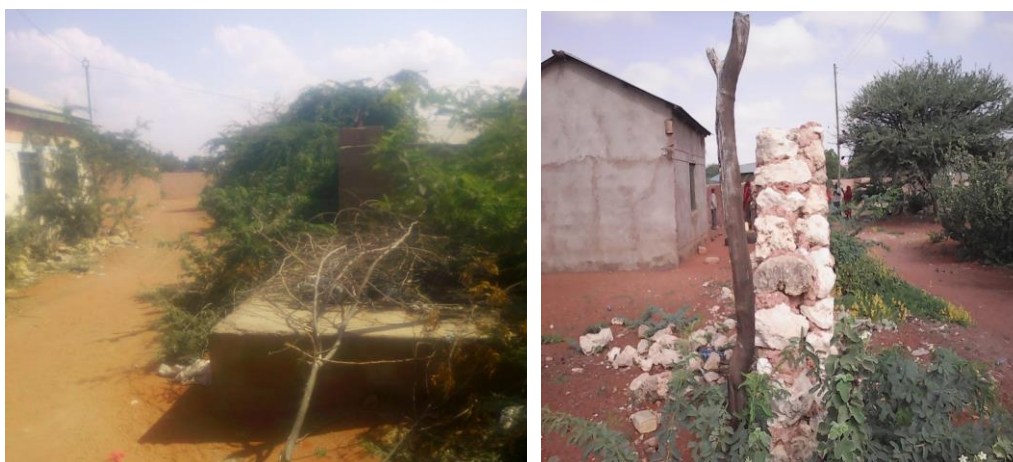
Figure 2-18: Septic Tank and Masonry Wall encroaching in Wagberi Location
