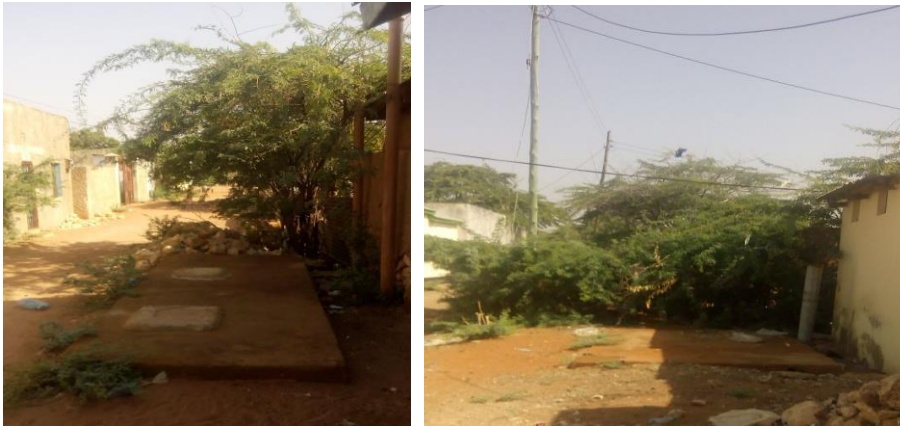
Figure 2-9: Septic Tanks encroachment on the Sanitary Lanes in Barwaquo Location
